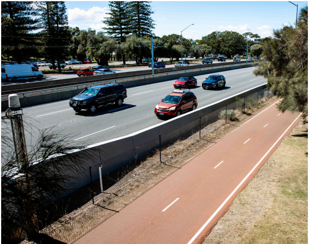
Path next to road with barriers
